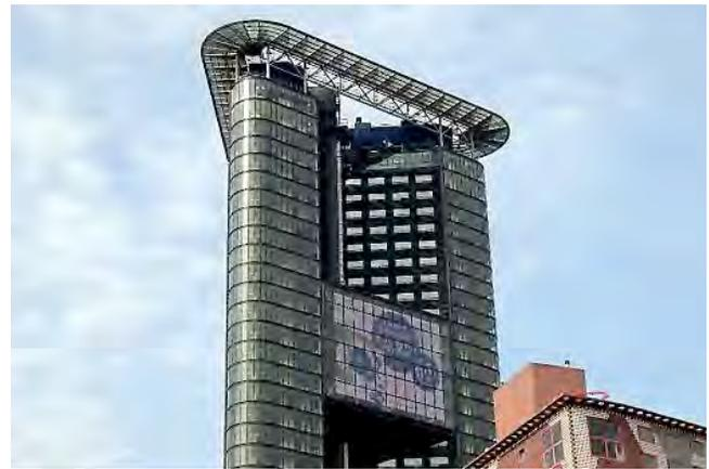
**Figure 5. Integrated LED screen mounted on *Het Strijkijzer* in The Hague.**
